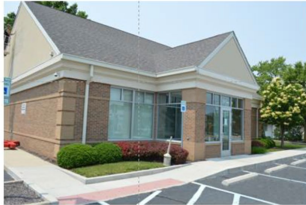
6410 N. College Avenue Site
