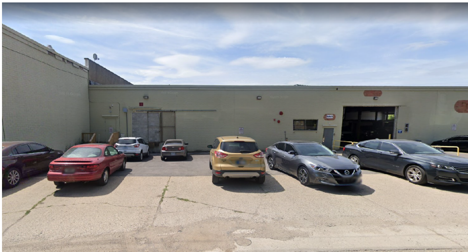
Figure II-1. Photograph of Existing Paratransit Facility
